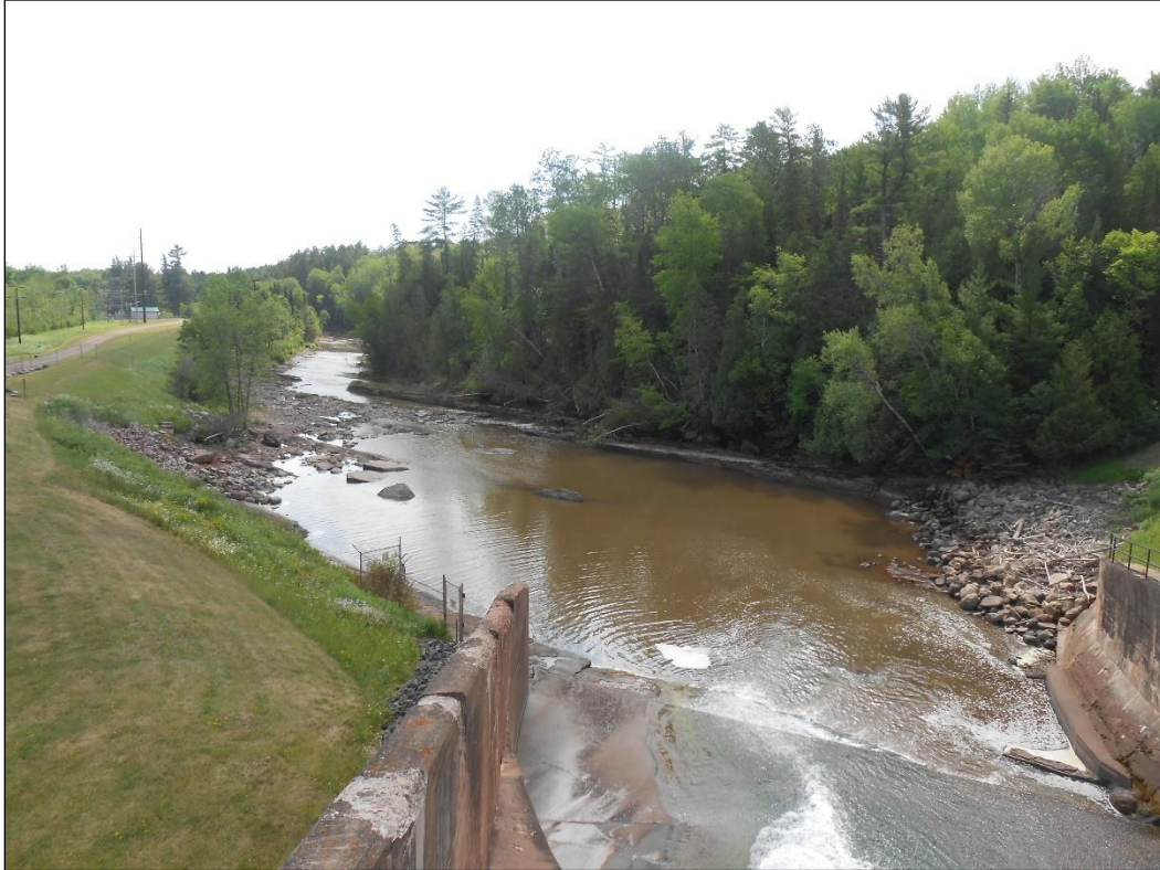
Figure 10.2-2 View downstream of the White River Dam (looking east)
