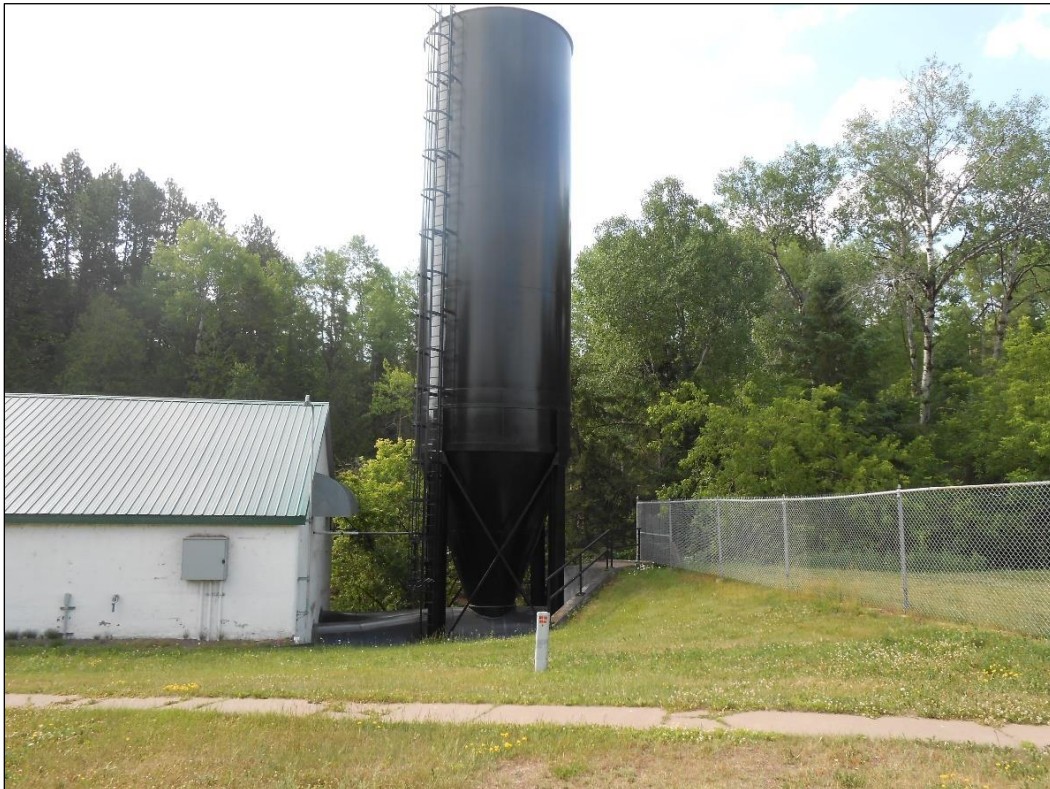
Figure 10.2-3 View of Powerhouse and Surge Tank (looking south)
