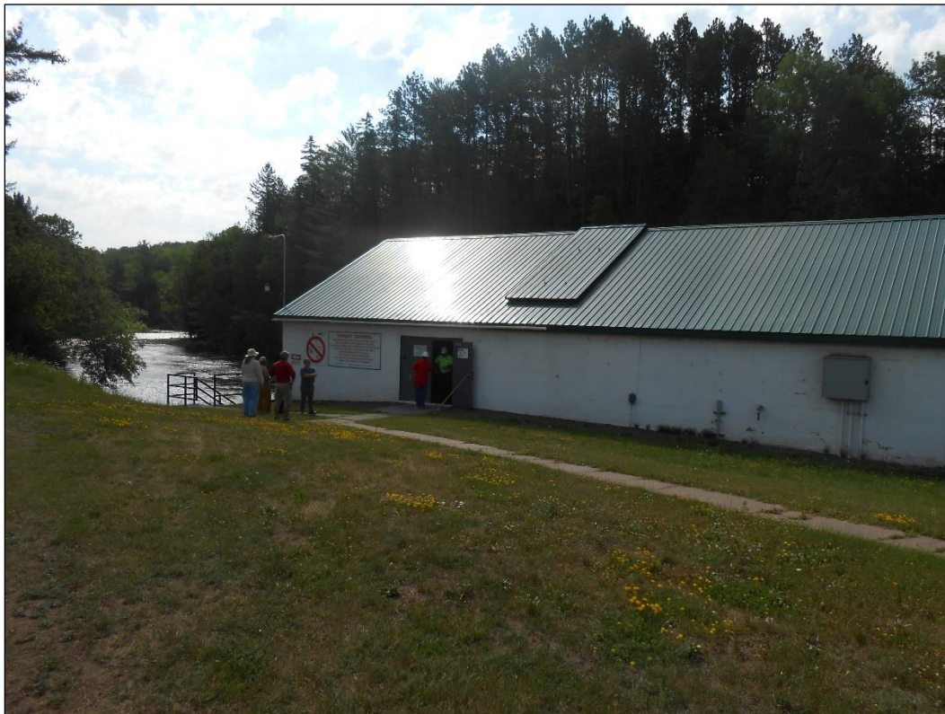
Figure 10.2-4 View of Powerhouse (looking southeast)
