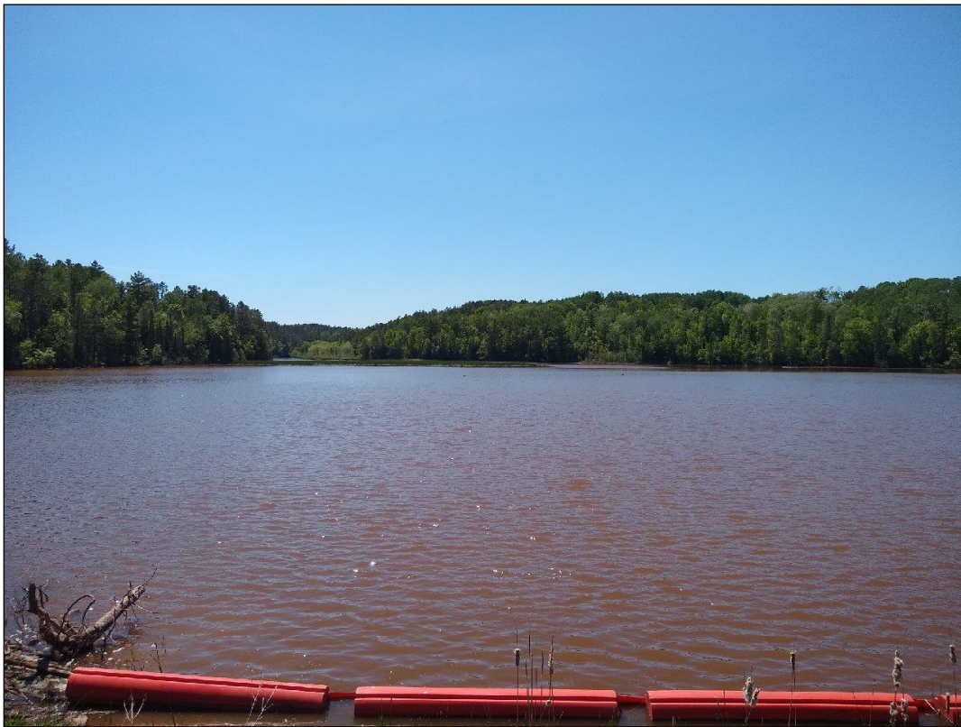
Figure 10.2-1 View Upstream of the White River Dam (looking west)
